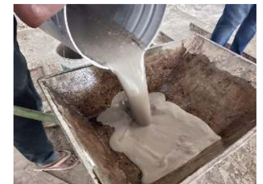
Placing the paste in moulds
