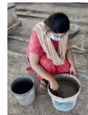
Mixing the materials
