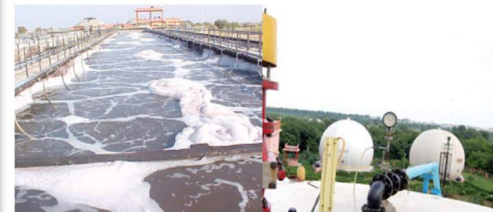
Aeration Tank in Function
