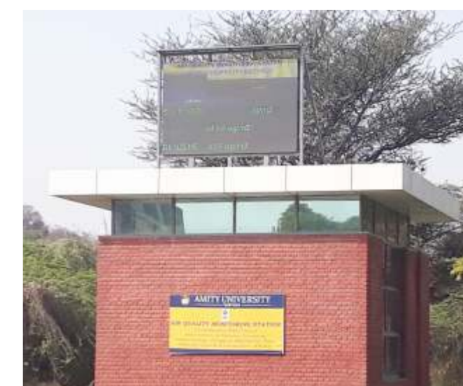
Side-view of Air Quality Monitoring Station (AQMS) at Amity University Haryana (AUH), Panchgaon Manesar Gurgaon.
