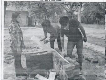
Cavity Wall -After every two layers 3 sheets of thermocol were stuffed in between the wall and butterfly ties were laid on the horizontal plane surface achieved
