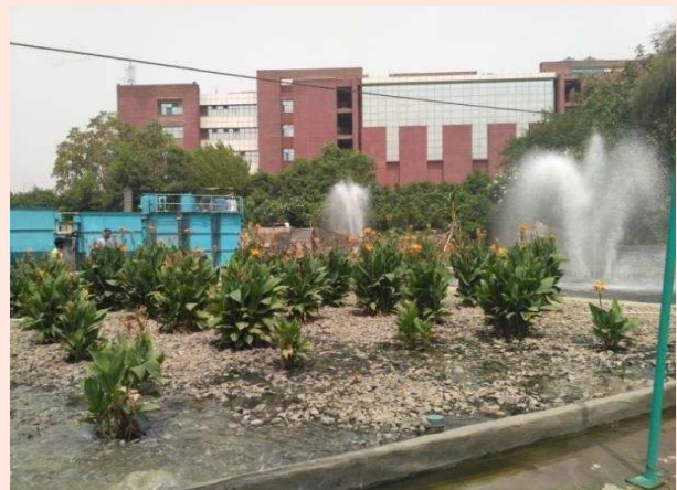
ETP Laundry Unit
