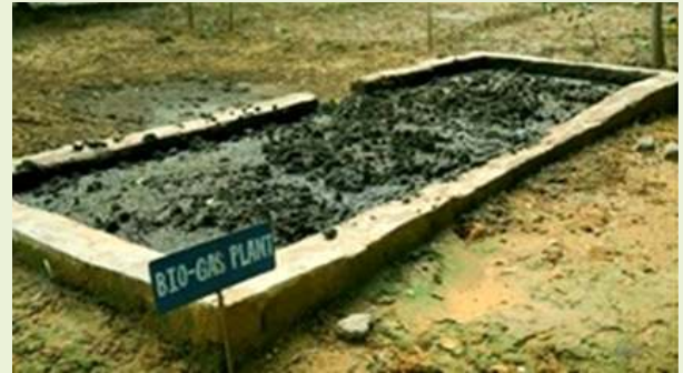
Biogas Plant at AUH
