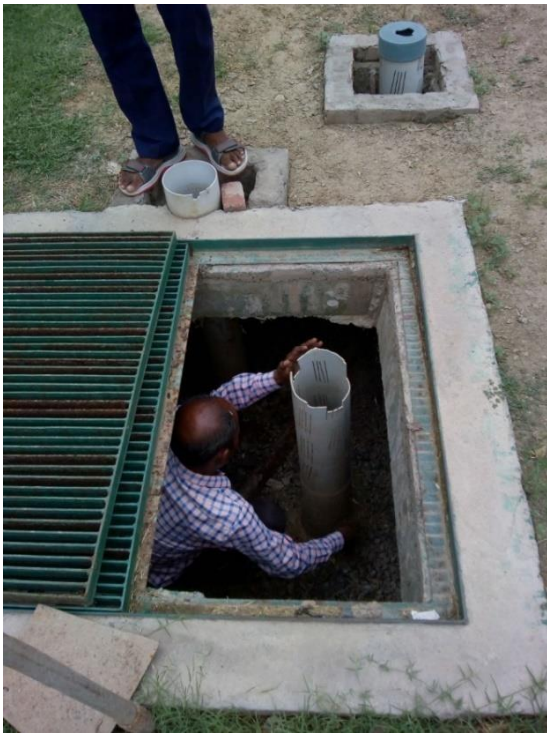
Maintenance of water harvesting structures before rainy season
