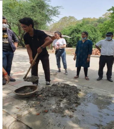
Preparation of mortar
