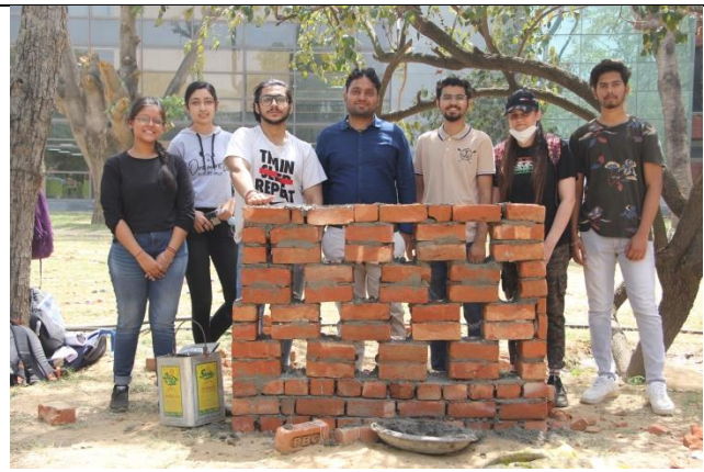
Completion of Jali
