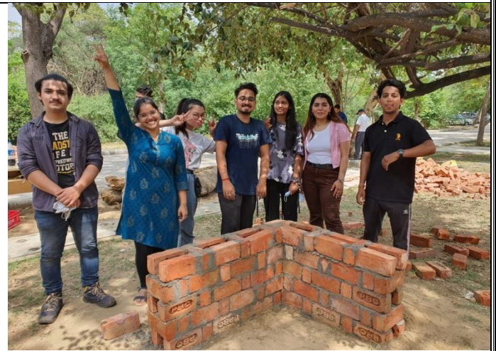
Completion of Rat Trap Bond
