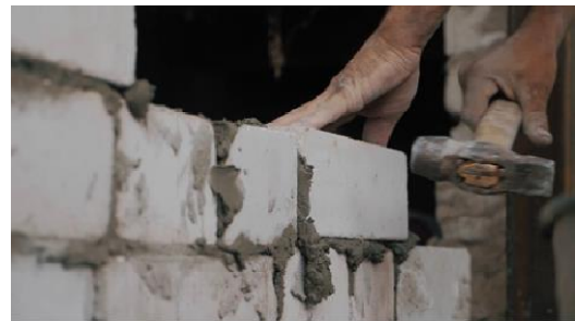
Fig. 1. Building up the Sample rooms with PCM embedded Bricks.
