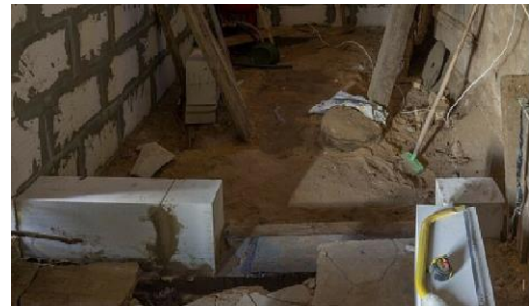
.Fig. 2. Image showing the masonry of the sample rooms
