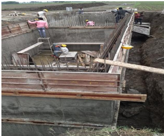
Fig.2. Existing Underground Water Tank (UGT)
