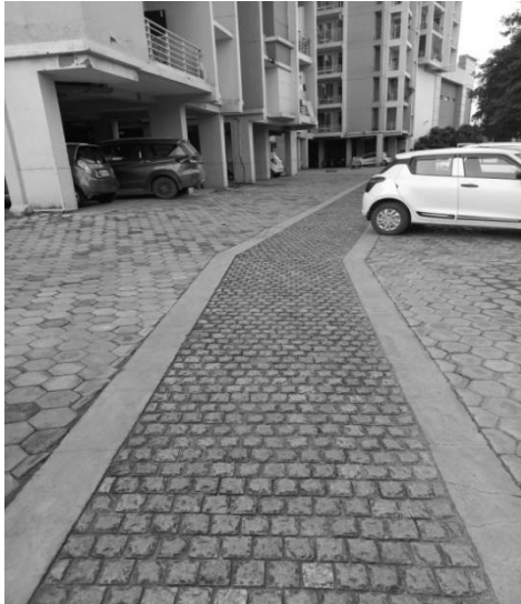
Figure 1: Paver blocks used in parking lots & in common space
