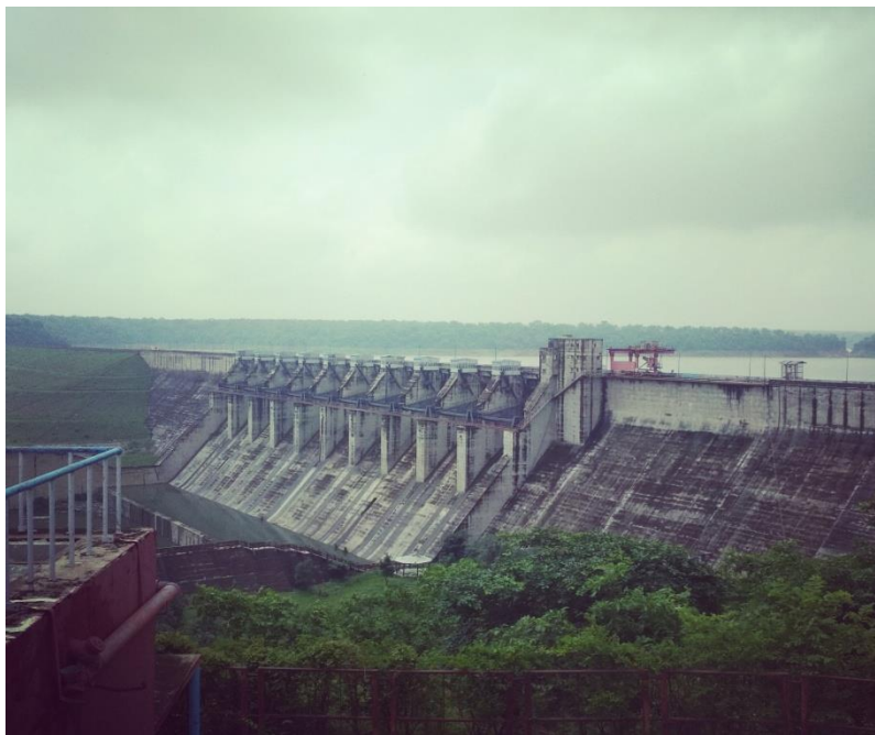
Figure 1: Madikheda dam, Shivpuri
