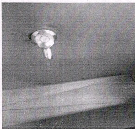
Fig. 2 A RO tap was leaking near Mechatronics lab on ground floor
