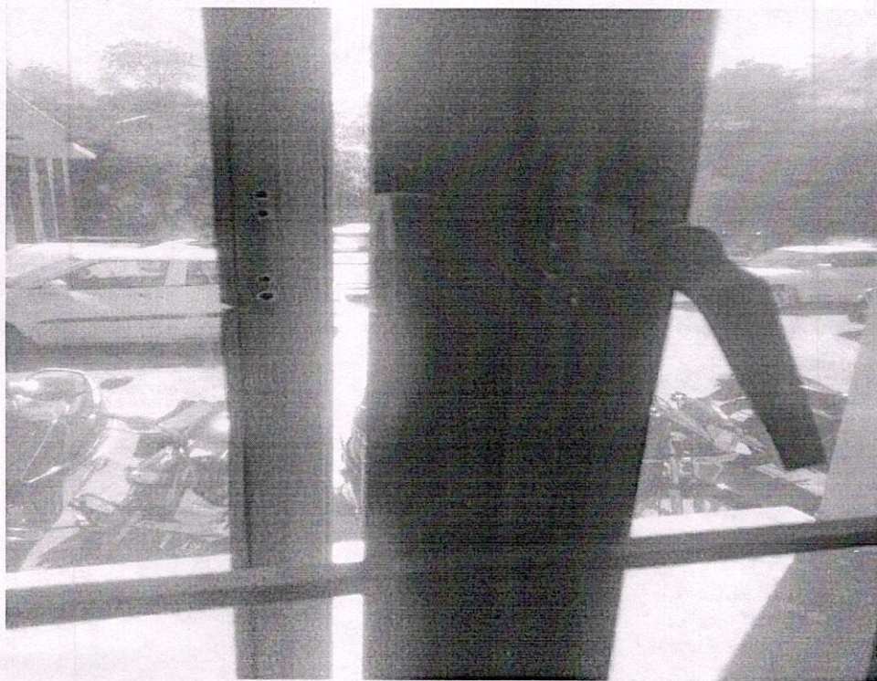
Fig. 3 In lab 112(B), a window handle is missing
