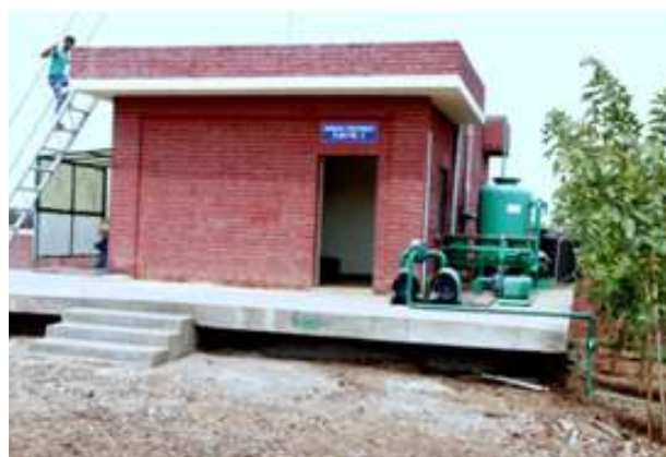
SEWAGE WATER TREATMENT PLANT – 2
