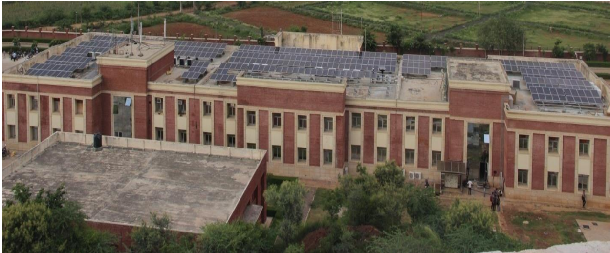
Rain Water Storage System
