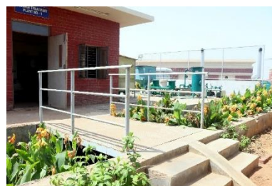
Sewage Treatment Plants (STP) at the campus
