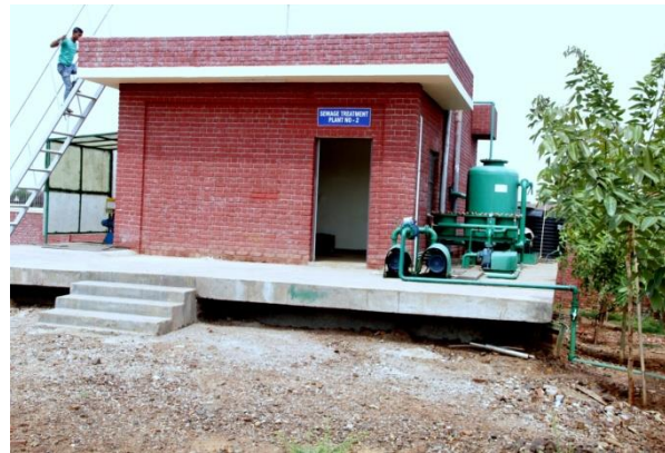
SEWAGE WATER TREATMENT PLANT – 2
