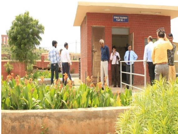
SEWAGE WATER TREATMENT PLANT – 1
