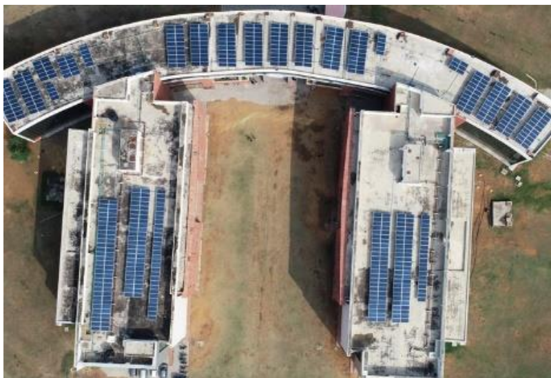
Solar Plant and dedicated Solar Park at Amity University Rajasthan
