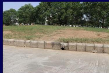
**Surface Drain Pipe (Side View)**
