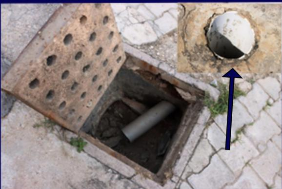
Surface Drain Pipe (Top View)
