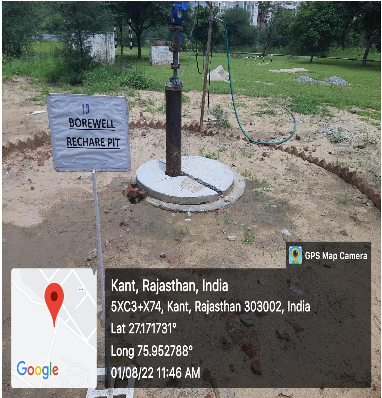
Borewell Recharge Pit-2
