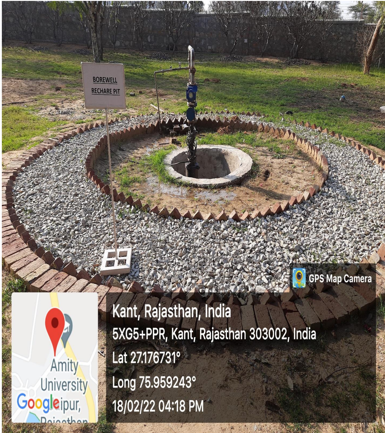
Borewell Recharge Pit-1
