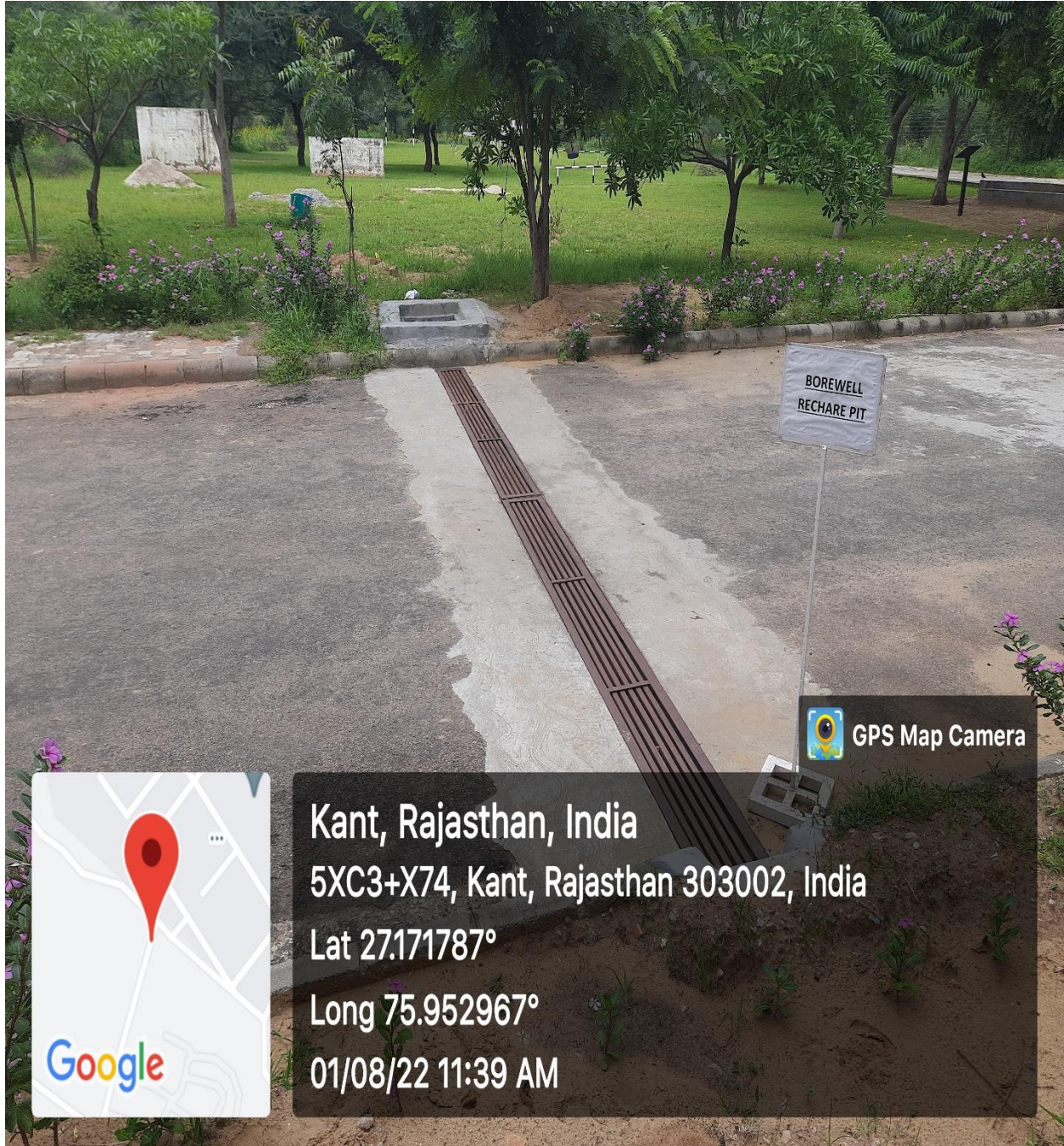
Borewell Recharge Pit-3
