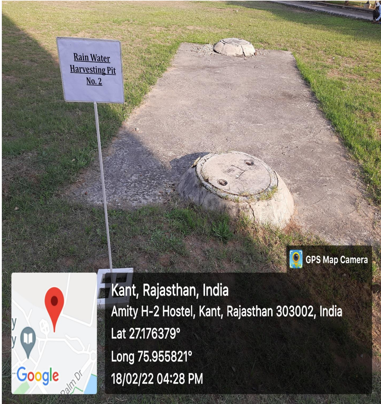
Rainwater Harvesting Pit No.-2
