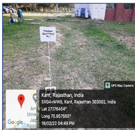
Rain Water Harvesting Through Recharge Pits at Amity University Rajasthan
