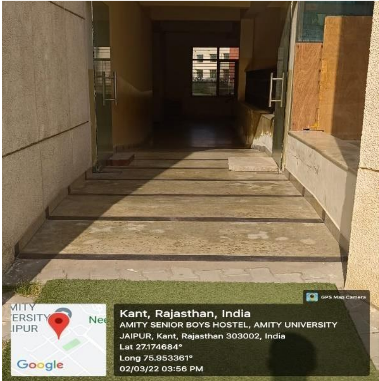
Ramp - Boys Hostel
