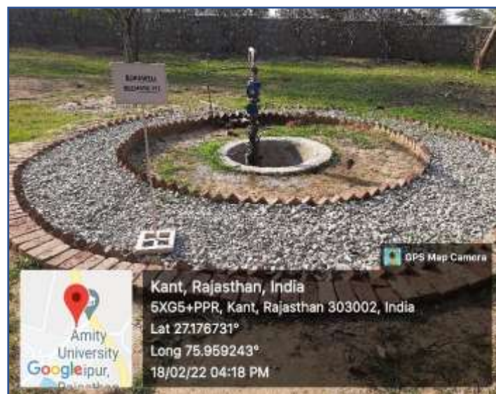
Rainwater flows into the recharge pit
