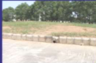
Surface Drain Pipe (Side View)
